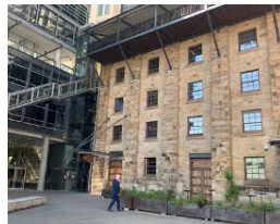
Figure 4-7: 1844 Australian Gas and Electricity Building, Hickson Rd (Source: Curio Projects 2020)
