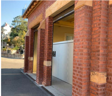
Sewerage Pumphouse, location of sign
