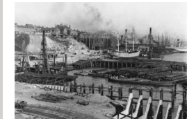
Figure 4-11: Millers Point towards gasworks c.1909 (Source: State Library NSW)
